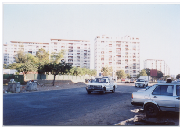
Coop-House where maintenance is becoming problematic
