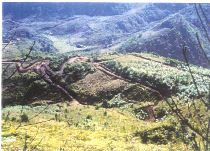
P. 1 View of F3 orebody from north-west
