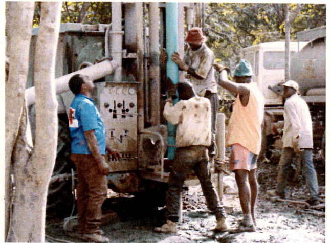
MJMB-E3: PVC casing is inserted.
