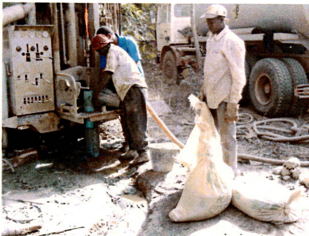
MJMB-E3: Gravel sand is inserted between bore hole and casing.
