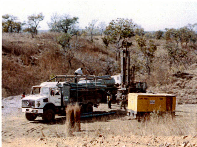
MJMB-E2: preparation for drilling
