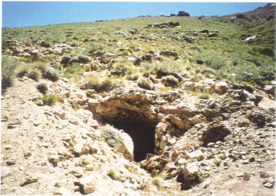
Plate 6 Varvarco district : A trench and drift entrance of Mina Santos located in the upper stream of Guaraco Norte creek
