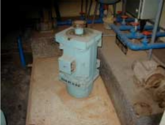
Removed Motor from Backwash Pump
