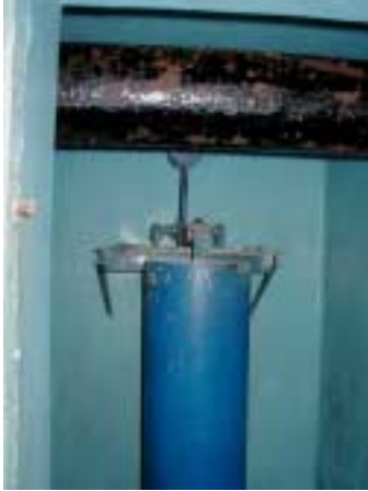
Filter Outlet Control Device (adjusting lever)
