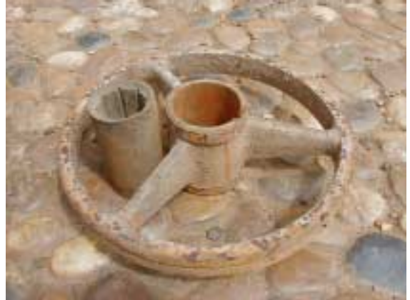
Support for Intermediate Pump Shaft (original support)
