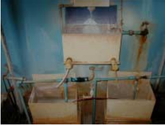
Hypo-chlorite Feeding Equipment (air intrusion into injector is observed due to drop of liquid level)
