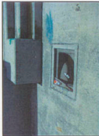
Photo-12 Lost Cover of Drain Pit
