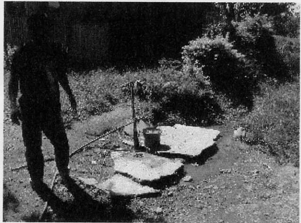
Existing Faucet(Dalacutan Area)
