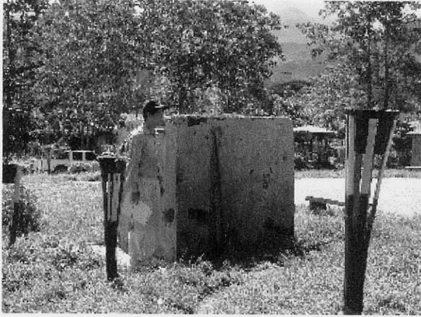
Reservoir Tank of Existing Level-2 System
