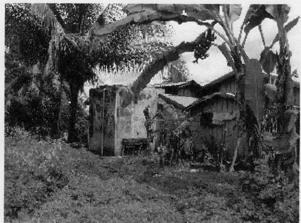
Reservoir Tank of Existing Level-2 System
