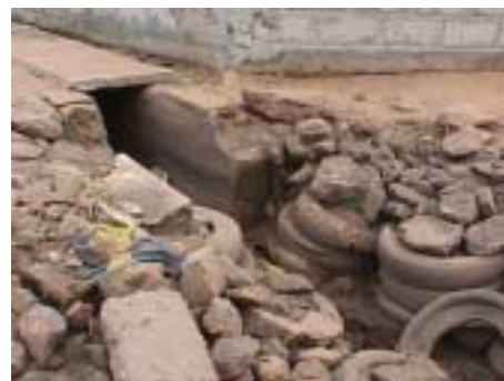
Road side gutters
