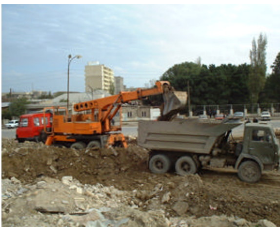
Cleanup Activities in progress
