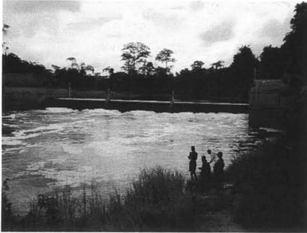
Agboville Existing Dam on Agneby River
