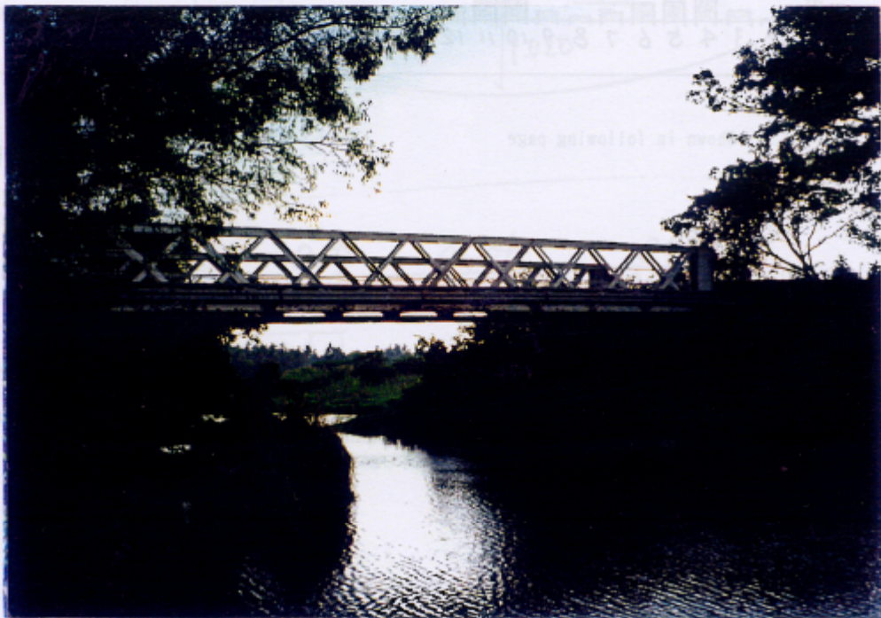
The side view (perpendicular direction to the bridge axis)
