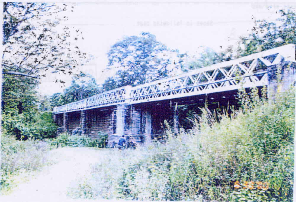
The side view (perpendicular direction to the bridge axis)
