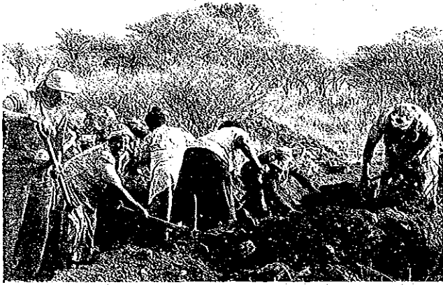
Women constructing water supply facilities as part of the "Plan for Expansion of the Magalies Water Supply Zone."
