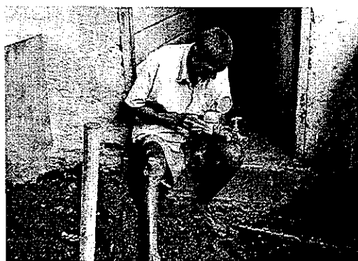
Giving an Individual Water Connection
