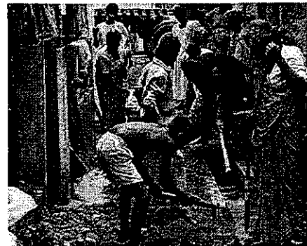
Beneficiary Families Engaged in Digging Trenches for Laying Service Lines in the Settlement
