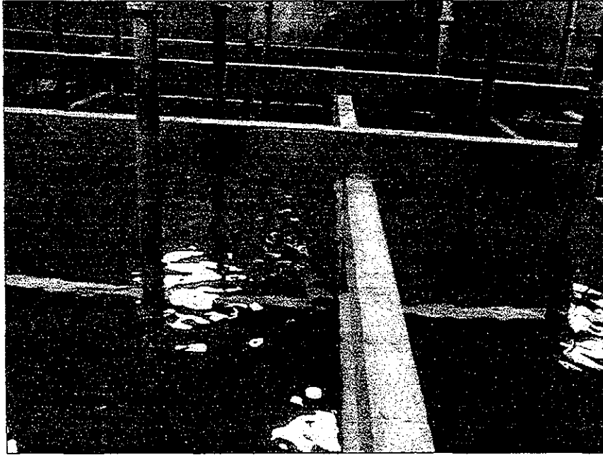
Photograph M1 – Wall Tie Beam Grid and Roof Columns
