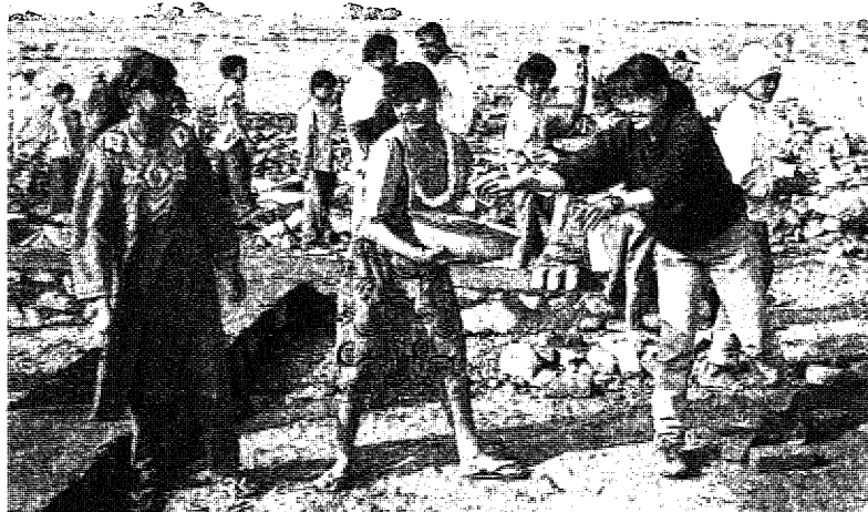
Paul Quayle "Japanese Volunteer Helps Construct a School" (国際協力フォトコンテストより)
