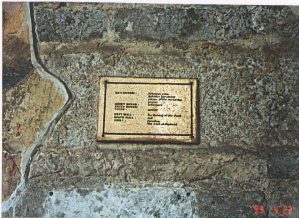
Metal sign board, giving minimal information in Turkish/English. All signs are too small, often rusting as is this one, and in most cases hung too high, making them almost illegible.
