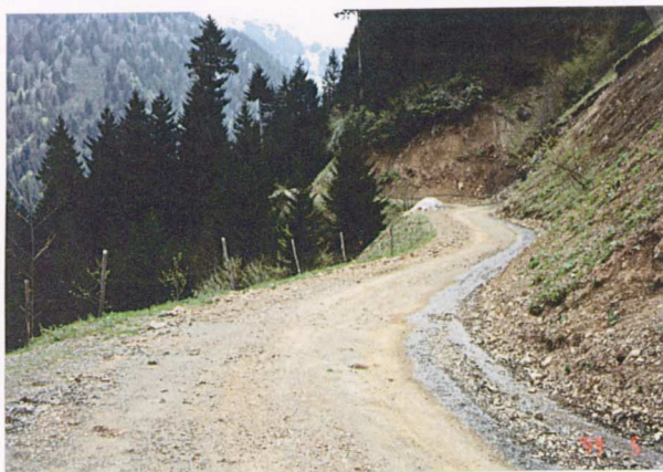
Access road to the panorama point. Need immediate improvement (surfacing, drainage, landscaping, etc.).
