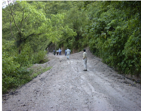
Photo 2.3.2 Landslips at Route 34
