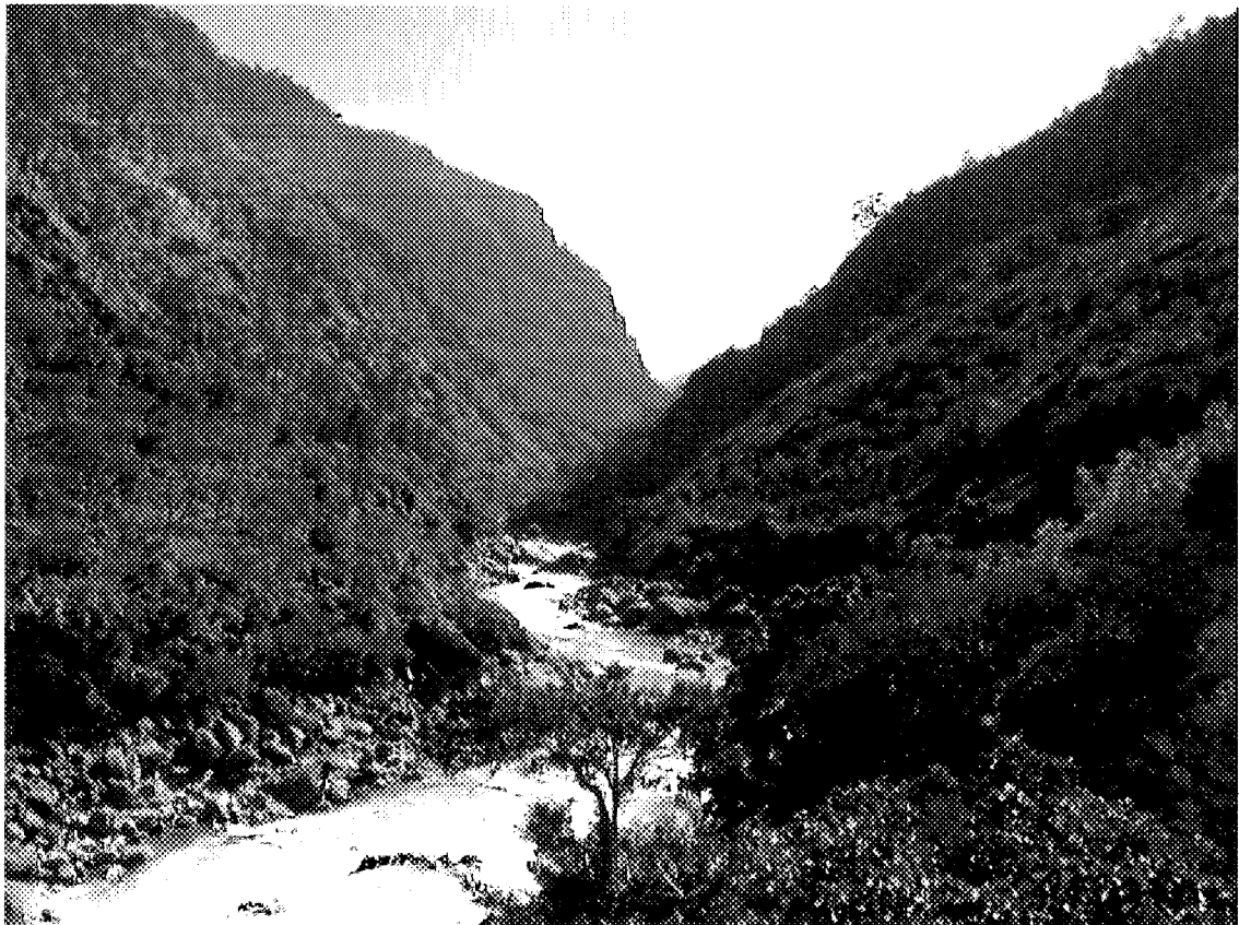
Upstream View from Dam Site (3.120)
