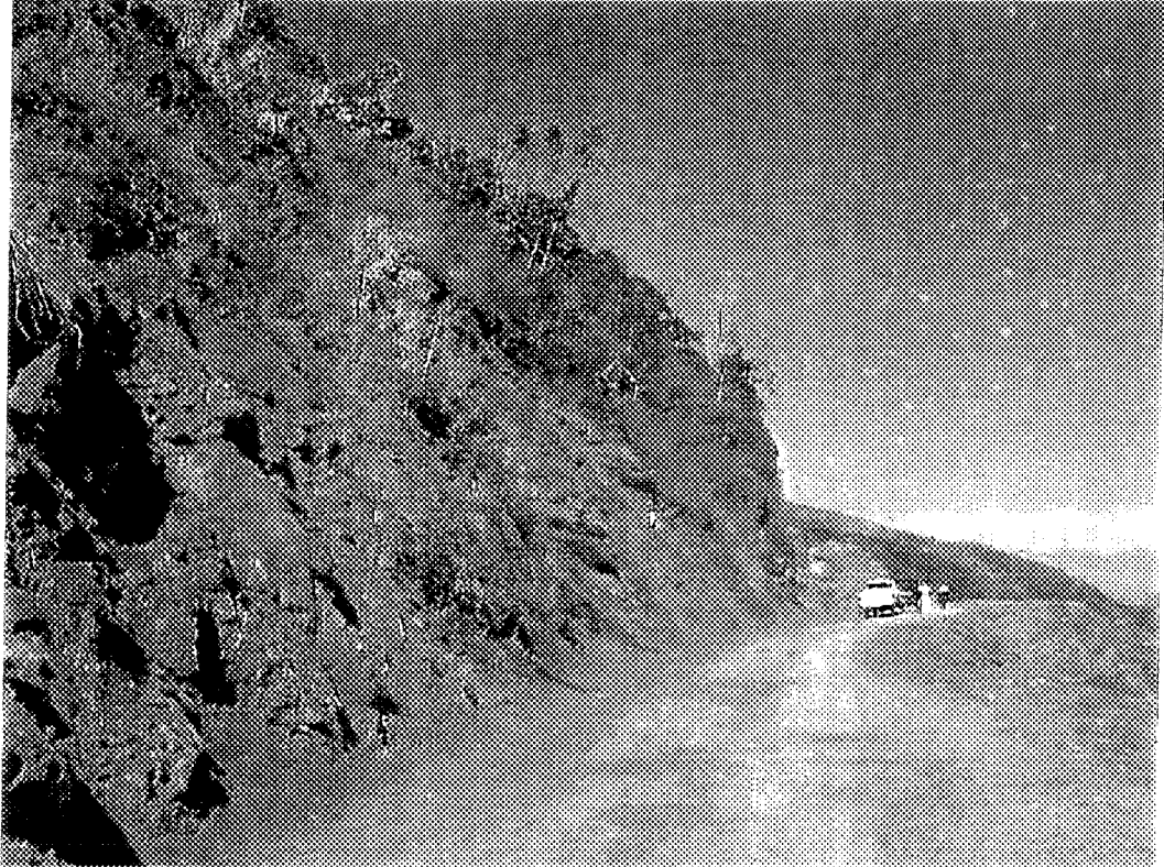
Road Condition at Dam Site
