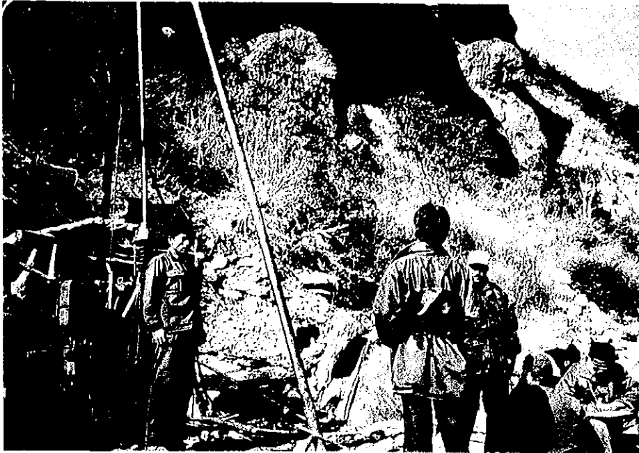
Drilling at Dam Site
