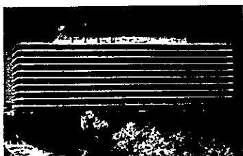
Kumamoto Prefecture Office Building
