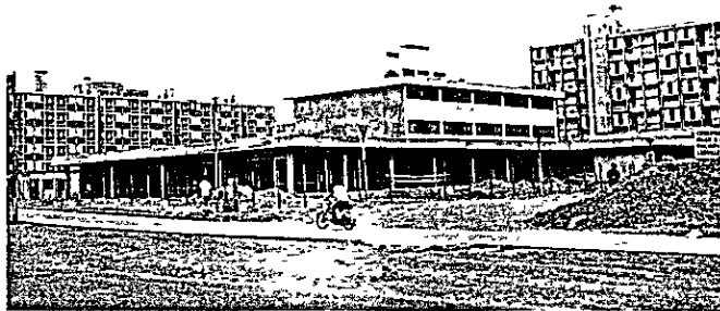
The first phase of construction of the Peruvian Japanese Cultural Center
