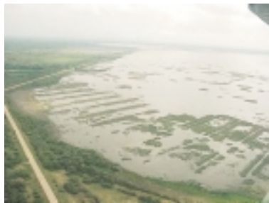
Lake Lubana near the Aiviekste sluice
