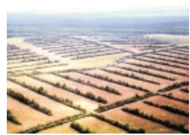
Drainage in Grivu
