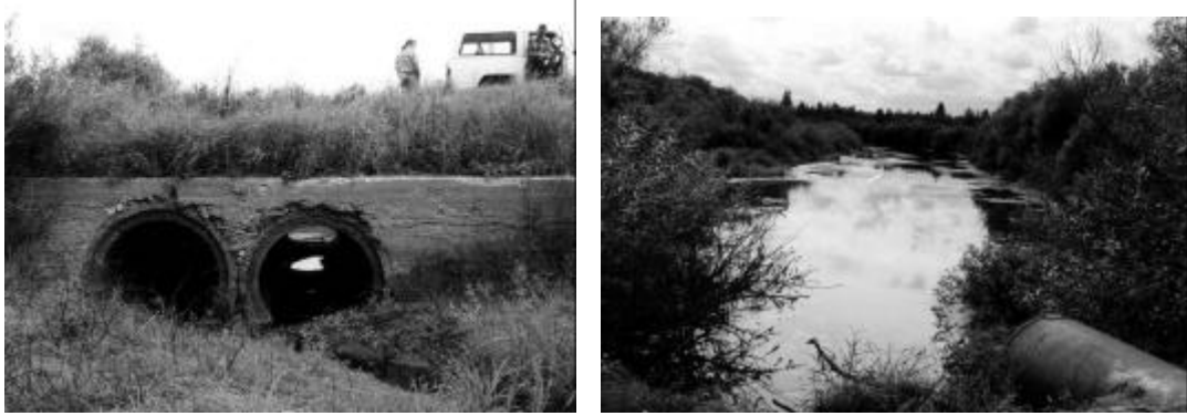
Culvert (left) at Fen Area (right).
