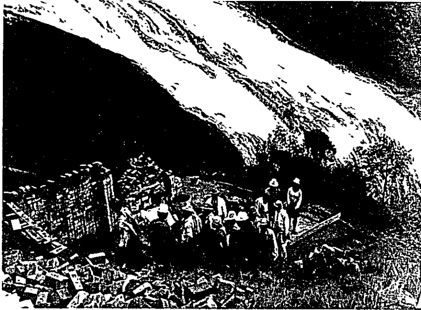
Small- scale hydroelectric plant (1) Constructing work for the small- scale hydroelectric power station (Analamihoatra village)
