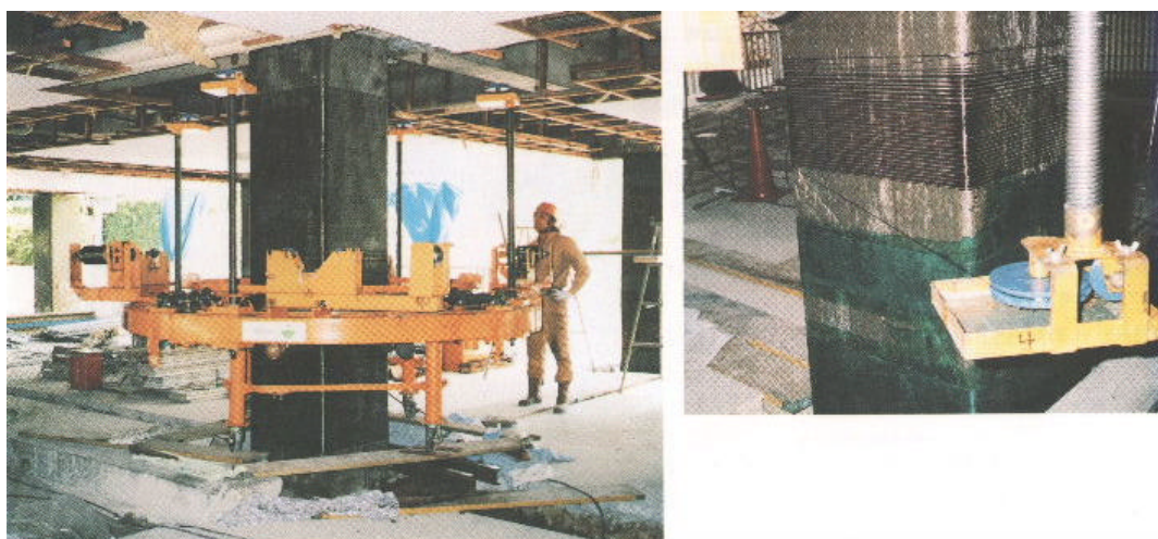
Figure 8.2.5 Carbon Fibre Lining
