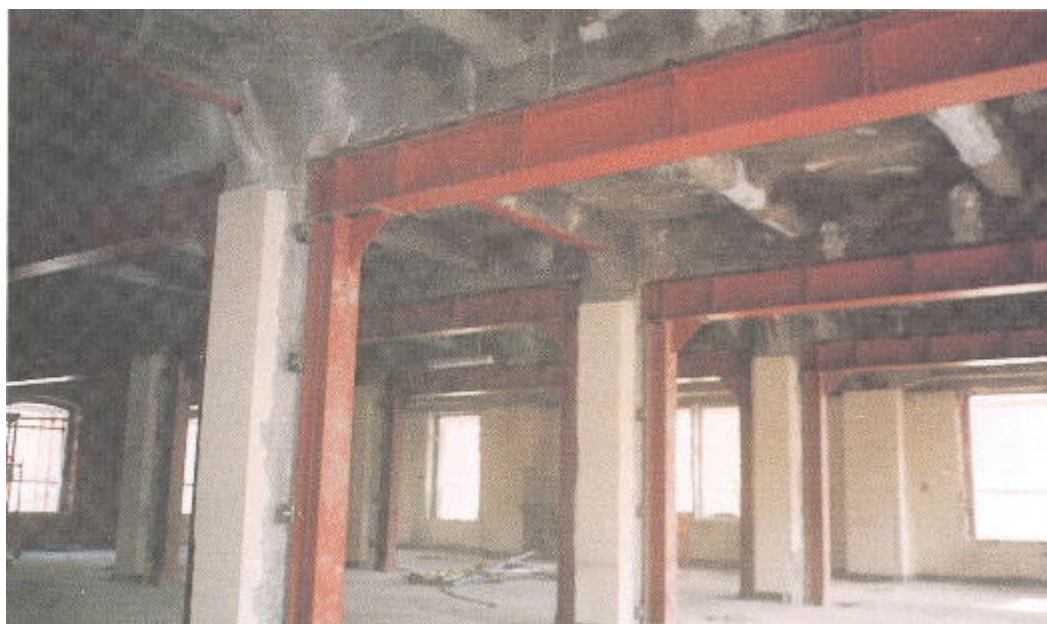
Figure 8.2.4 Reinforcement of Columns and Beams
