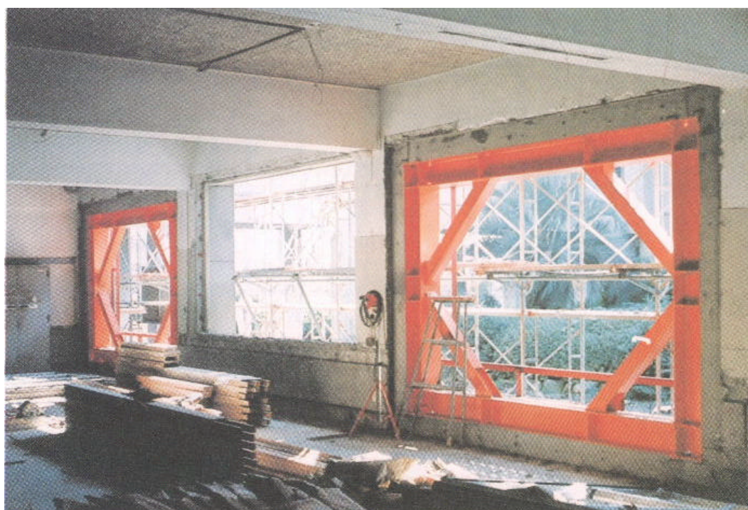
Figure 8.2.1 Steel Bracing Added to a School Building
