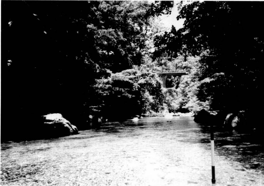
Photo 5-7-12 Downstream Area of Kware'a Dam.
