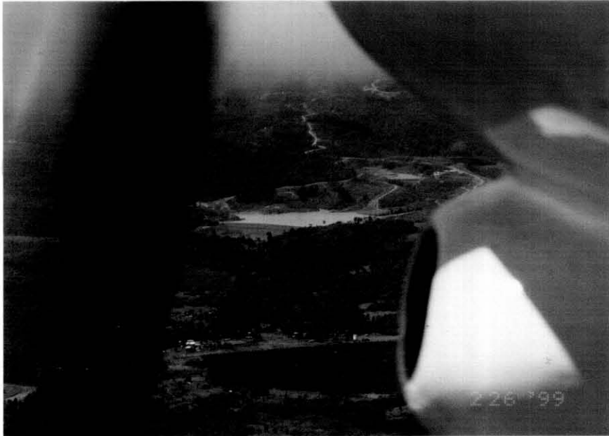
Photo 5-7-1 Gold Ridge Access Road (Maotapuku 1,2)
