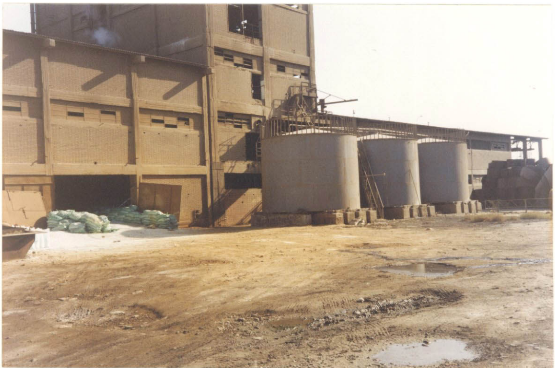
Photo. EIS-6 Building for Spent Sulfuric Acid Recovery Unit Left: By-product Ferrous Sulfate Bags Right: Fresh Sulfuric Acid Tanks
