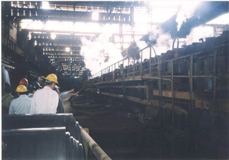
Photo. EIS-1 Pickling Plant at Cold Rolling Mill Facility
