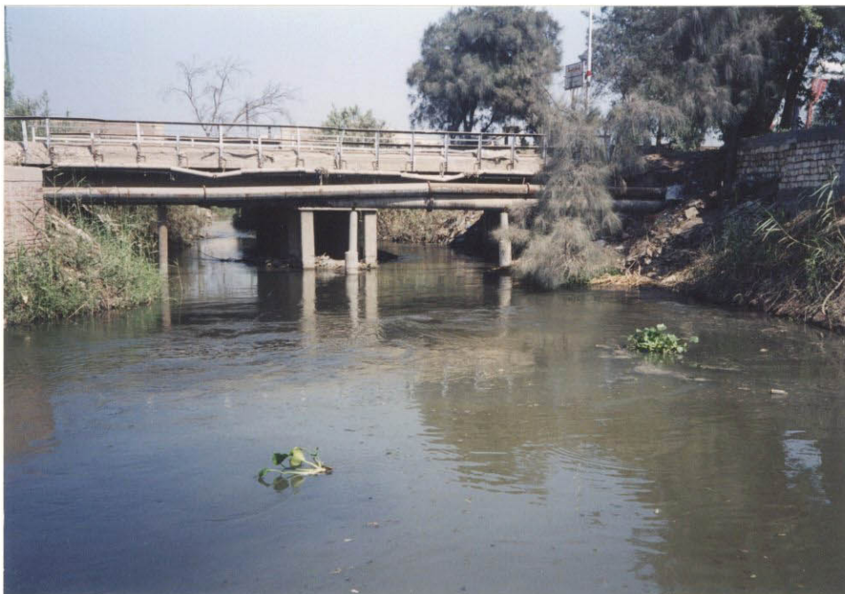
Photo. MRC-4 Non Potable Water Canal trough Industrial District
