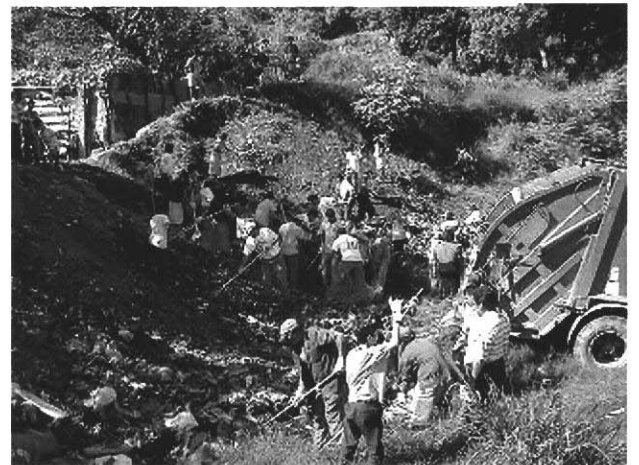
The suitability of the container collection system in marginal areas where collection is unsatisfactory was studied. The clean-up operations were carried out to encourage the residents to dump waste into the containers.
