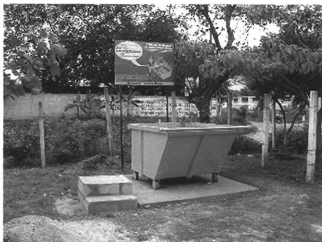
Containers were made and installed in the pilot project areas where waste collection is not satisfactorily provided.
