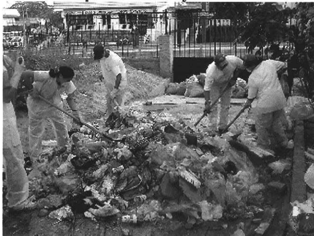
Thorough mixing of collected waste samples
