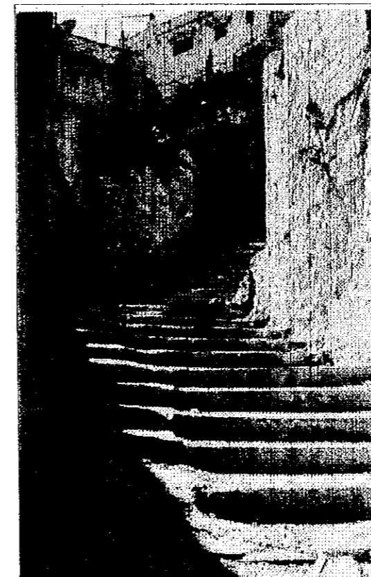
PAINT THE CONCRETE WALL WITH SUITABLE COLOR AND REMOVE ELECTRIC WIRES
