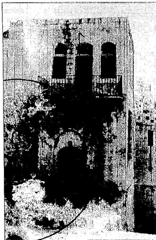
CLEAN THE STONE AND MAINTAIN THE ENTRANCE DOOR & REGLAZE THE WINDOWS. REMOVE EXTRA SOIL. EMPHISISE ON THE HISTORICAL ELEMENT IN THE SITE (TREE, DOOR, ... ETC.)
