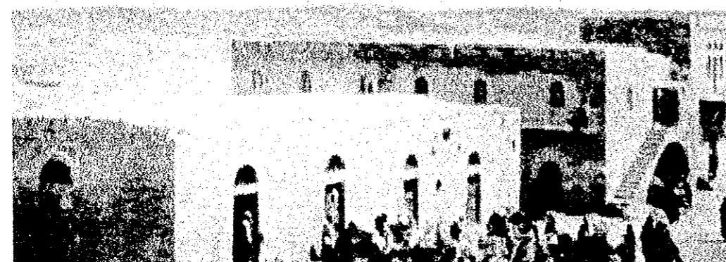
PHOTO NO. (3) AL-SHAMAYLEH BUILDING EARLY TWENTIETH CENTURY
