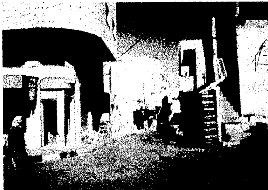
PHOTO NO. (32A)
