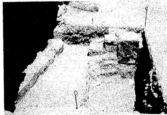
SOUNDINGS & EXCAVATIONS (MUSEUM PLAZA) PHOTO (7)
