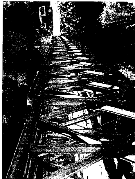
Main beam was bent and rusty.
