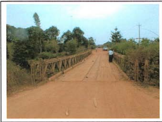
Picture 1 : Existing bridge
