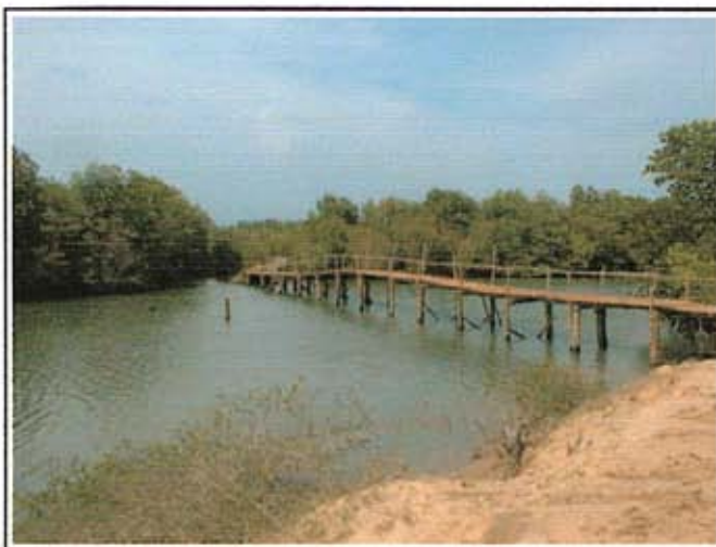
Picture 1 : Temporary bridge
