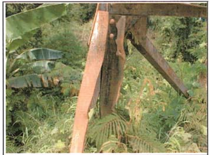
Picture 2 : Existing bridge
