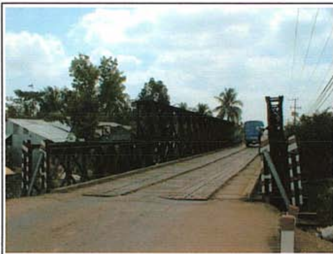
Picture 1 : Existing bridge
