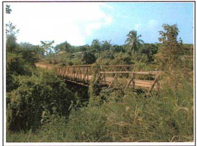
Picture 2: Existing bridge
