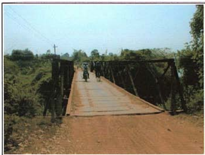
Picture 1 : Existing bridge
