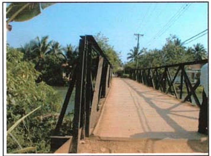
Picture 2 : Existing bridge
