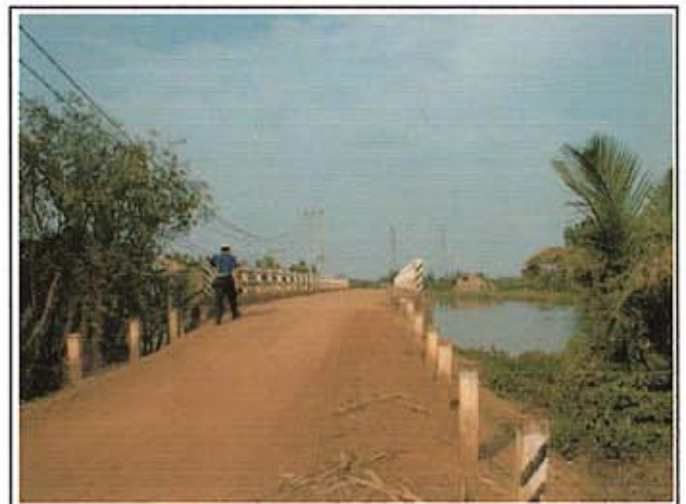
Picture 2 : Existing bridge
