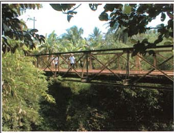
Picture 1 : Existing bridge
