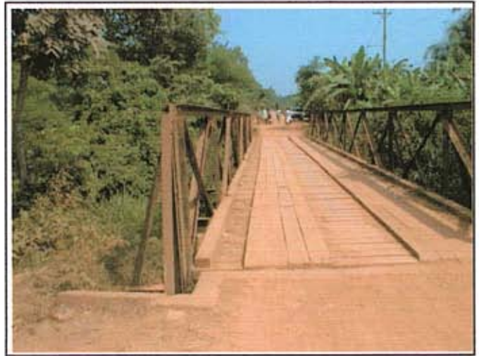
Picture 2 : Existing bridge
