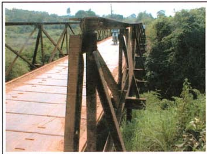
Picture 2 : Existing bridge
