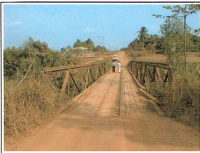
Picture 1 : Existing bridge
