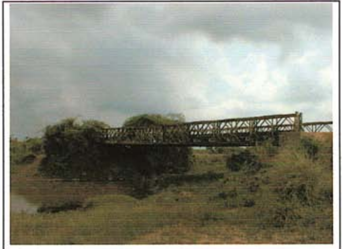
Picture 2 : Existing bridge
