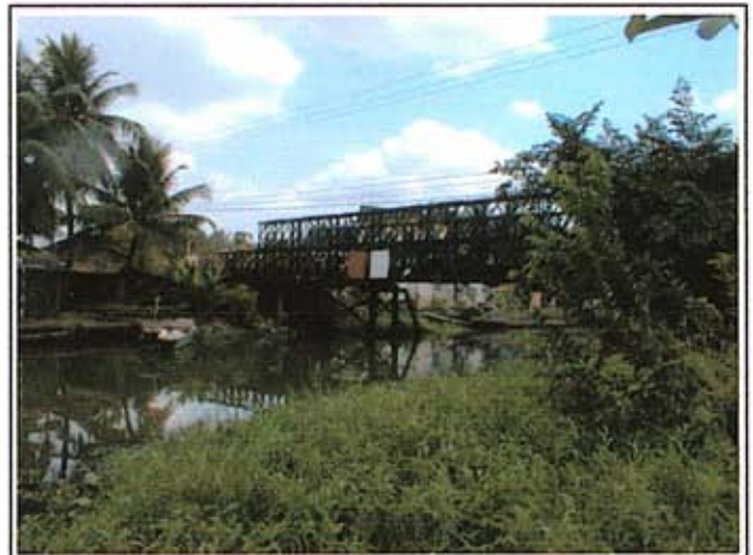
Picture 2 : Existing bridge
