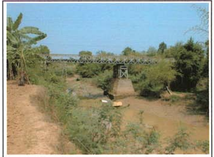
Picture 2: Existing bridge
