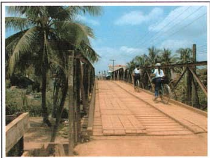
Picture 1 : Existing bridge
