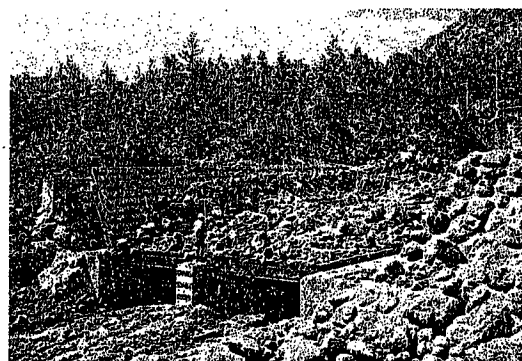
Trapped Debris Materials on Screen
