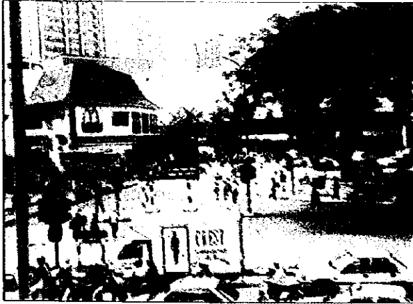
Intersection at Jalan Cheng Lock and Jalan Sultan
