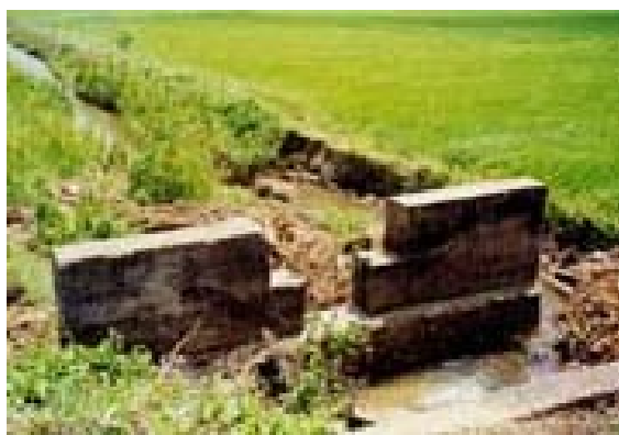
Erosion at Turnout
