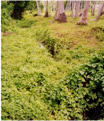
Distributary Canal (Poor Maintenance)
