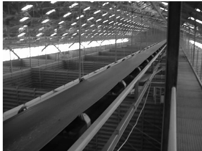
< Whole view of Cao Lanh Silo (Left) and a conveyor over the top of storage bins (Above) >
