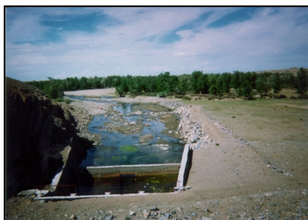
Photo I.10.7-2 Baruunturuun Power Plant Site
