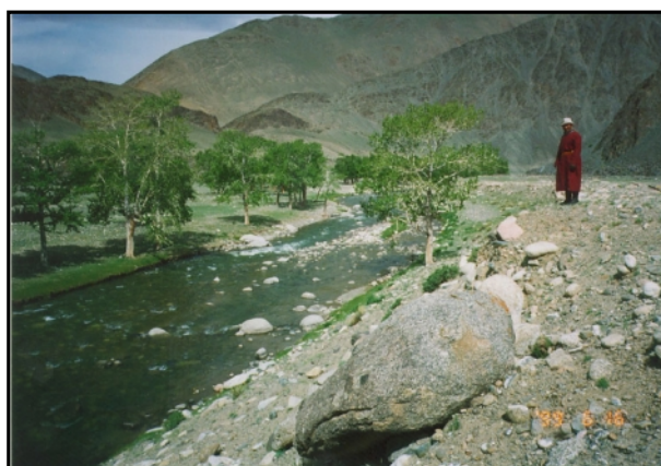
Photo I.10.7-1 Monkhaikhan Power Plant Site
