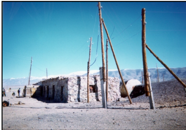
Photo I.7.5-1 Low Voltage Distribution Lines in Tolbo Sum of Bayan-Ulgii Aimag
