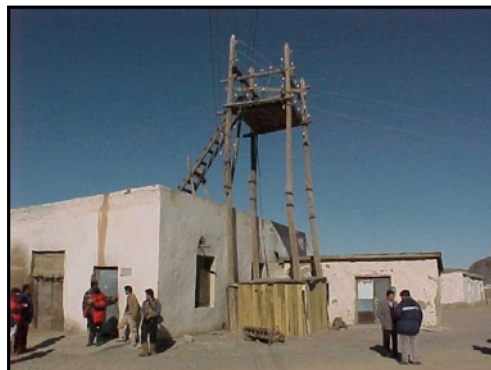
Photo I. 7. 4-1 Power Station Building in Mankhan Sum Center
