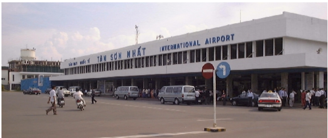
Photo 3.4.5 Passenger Terminal Building (Tan Son Nhat Airport)
