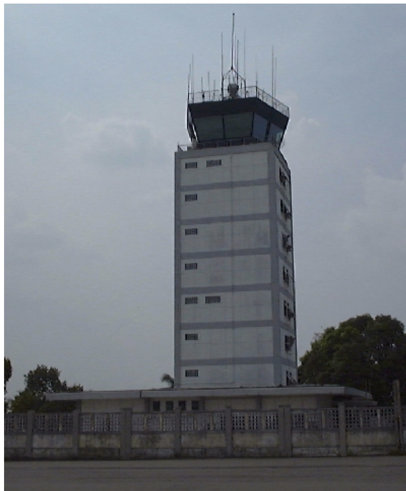
Photo 3.4.6 Control Tower (Tan Son Nhat Airport)
