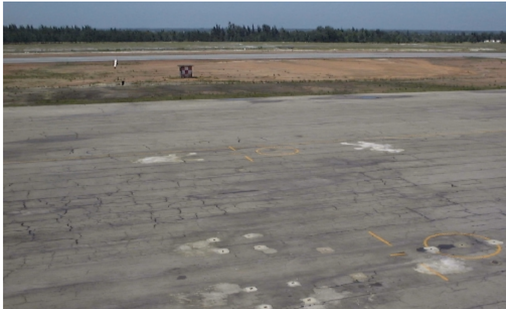
Photo 3.4.8 Apron Pavement (Phu Bai Airport)
