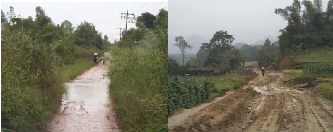
Figure 5.3.2 Existing Condition of Tertiary and Local Roads
