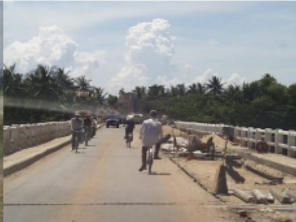
National Highway No. 1A Quang Ngai Province: Bridge Construction
