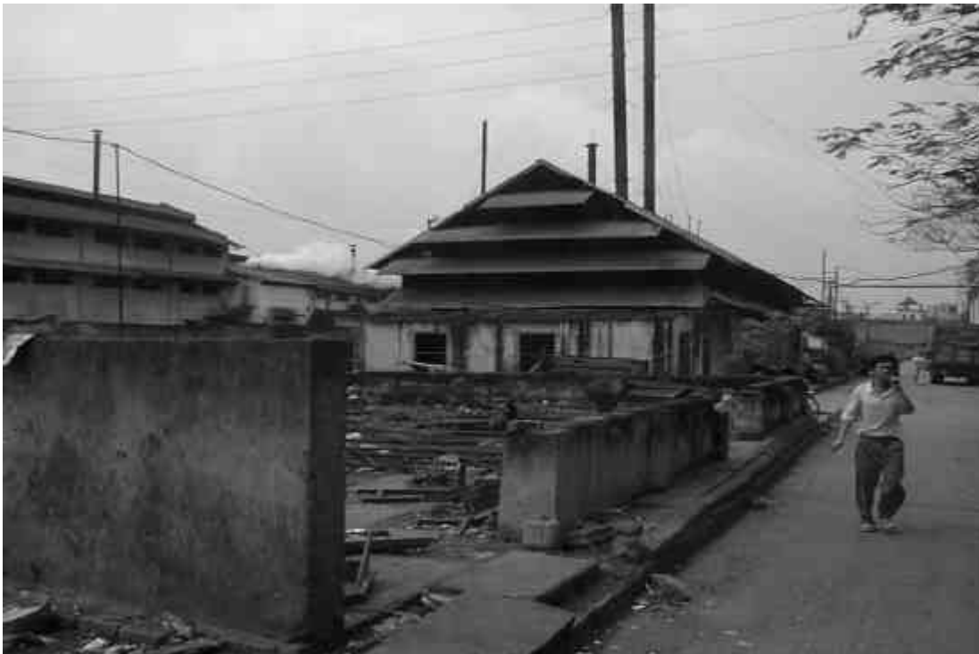
Figure 5 Site for a Wastewater Treatment System
