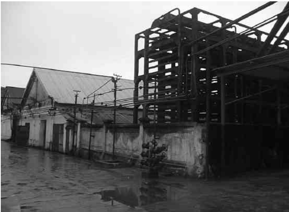
Figure 5 Wastewater Treatment System Site
