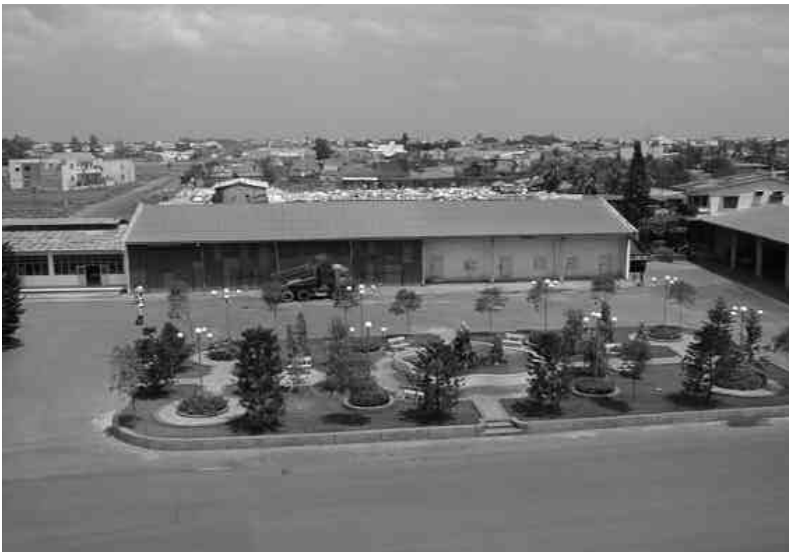
Figure 4 Site Planned for the Wastewater Treatment System
