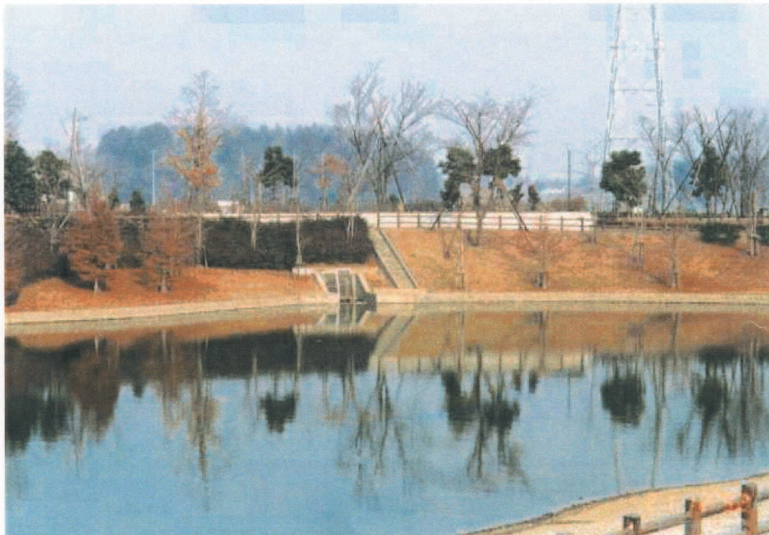
Outlet of Kasumigaseki Detention Pond
