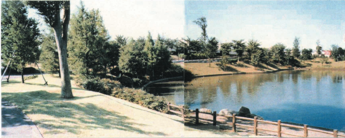
Kasumigaseki Detention Pond, Kawagoe City, Saitama (Built in 1990)
