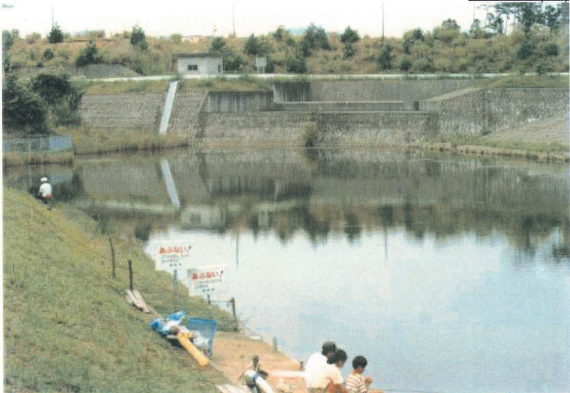
Kurokawa-II Detention Pond, Nagaoka City, Niigata (Built in 1982)
