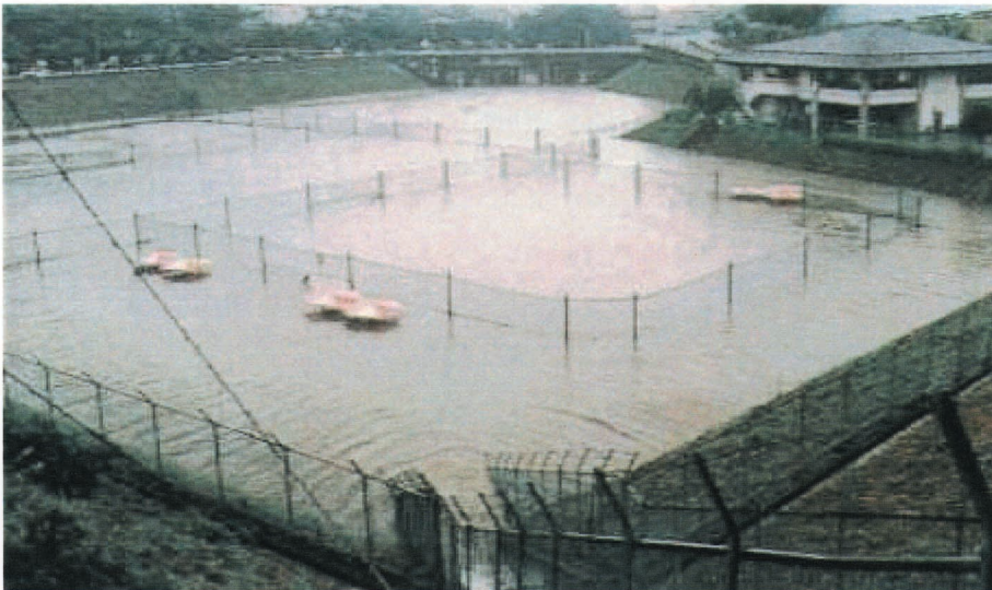
After Heavy Rainfall
